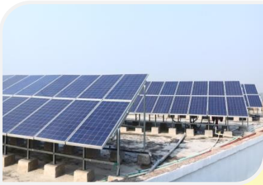
1. Solar generation Installation of Solar panels
